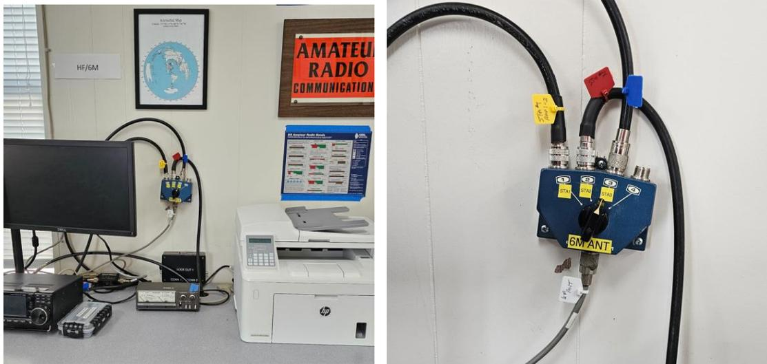
Antenna #1 position connects to antenna #2 of amplifier #1 (Station #1). Antenna position #2 connects to antenna #2 of amplifier #2 (Station #2), and antenna position #3 connects to the antenna port of station #3 IC-7300.
